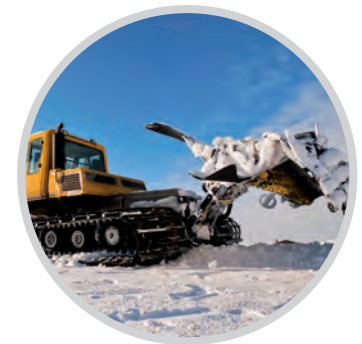
Ski area & high alpine construction
