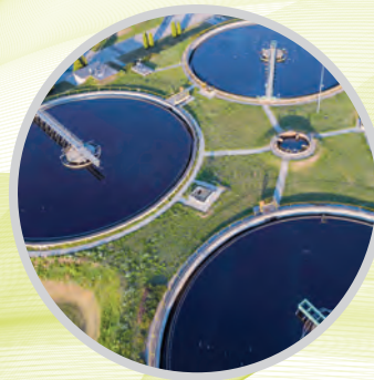
Sewage & waste water technology
