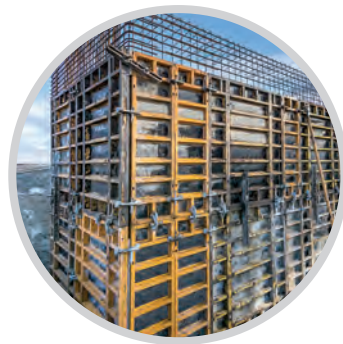
Building construction & underground engineering
