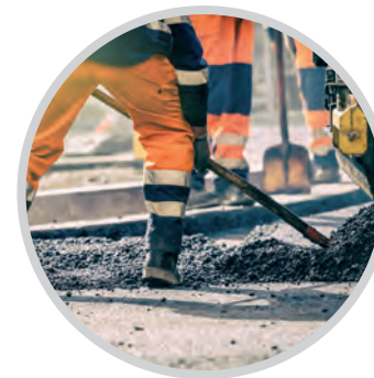
Civil engineering & road construction
